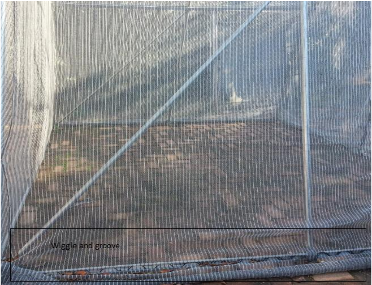
Common mistakes: Wobble and groove is installed wrong because its on the outside of the arch
